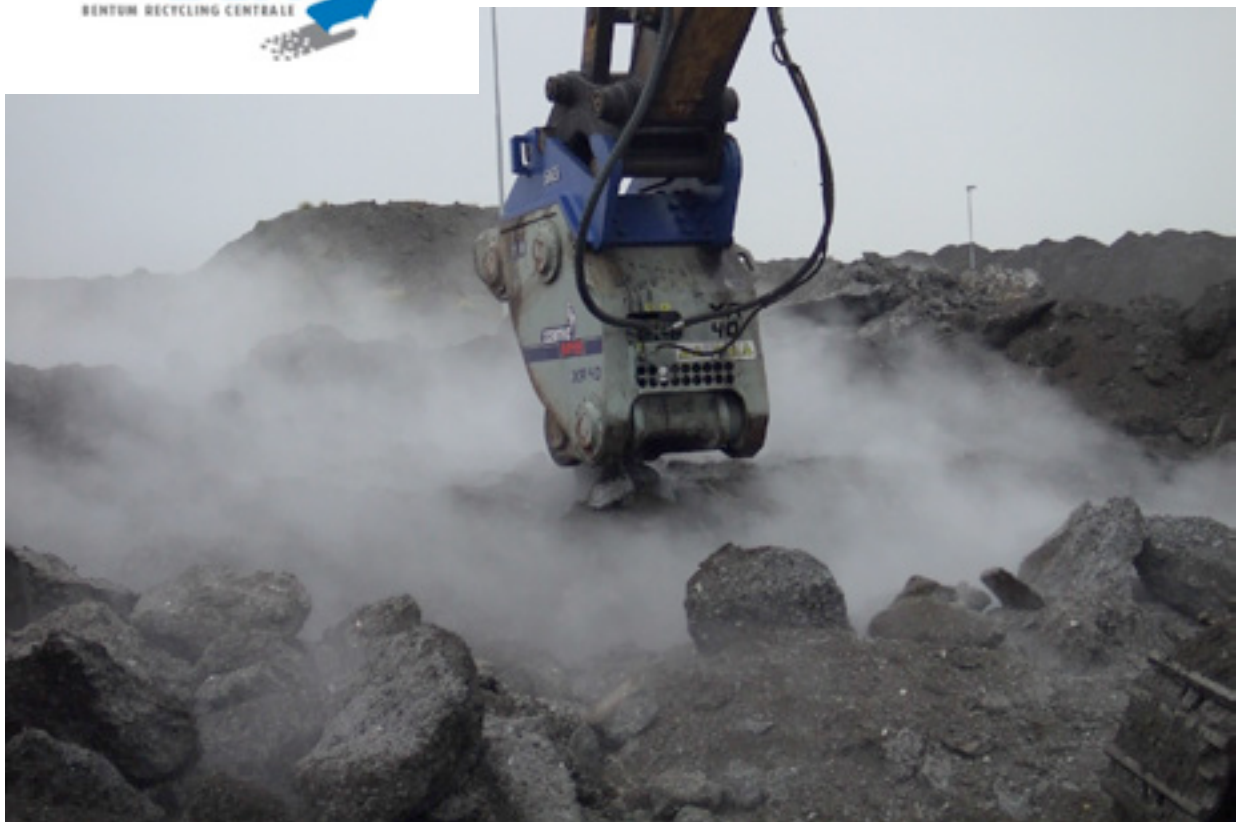
Model: XR40 – Project: excavating garbage incinerator slags in Amsterdam, October 2012
